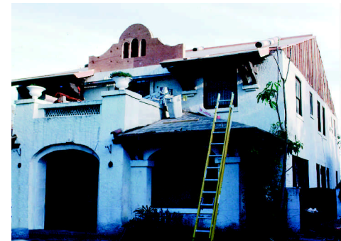
C: Reconstruction of original roof design in progress 1986
