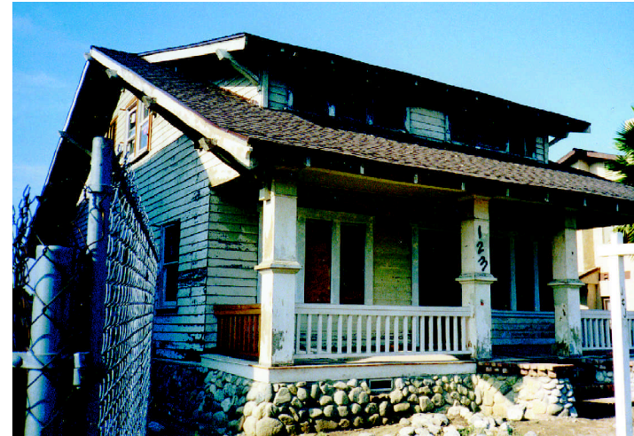
Historic house in the Kroeger/Melrose District saved from demolition and preserved as single family home. Relocated from 308 N. Olive Street for renovation.
