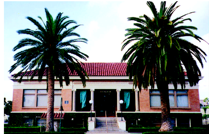
Former Carnegie Library now Anaheim Museum 241 S. Anaheim Boulevard (1908)
