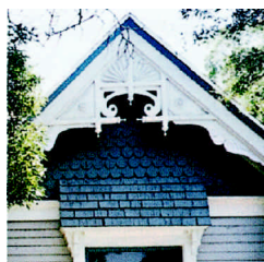
Appropriate historic detailing
