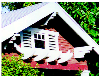
Preserved wood brackets
