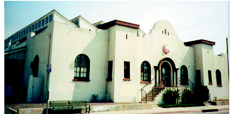
Citrus packing house at 454 S. Anaheim Boulevard (1919)
