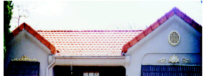
Original Terra-Cotta roofline with gutters and downspouts
