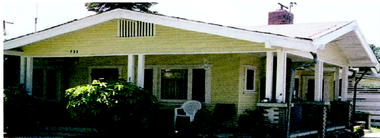
Porch with quoin design piers
