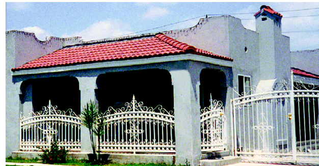
Inappropriate ornamental alterations
