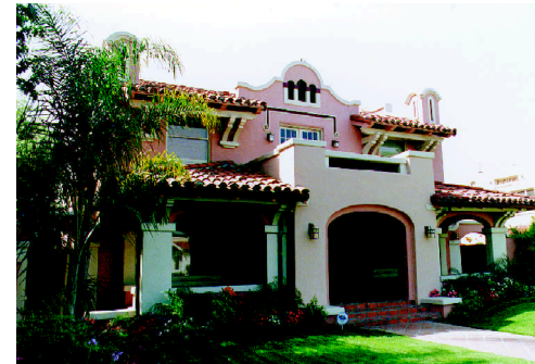
D: Exterior reconstruction completed in 1988
